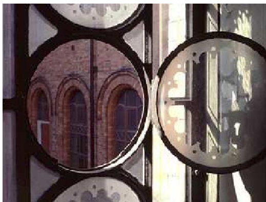
Window from the 1880s with etched glass and case-ment with openable vent made of cast iron in the old National Archive, Sweden. Photo Rolf Helmers.
