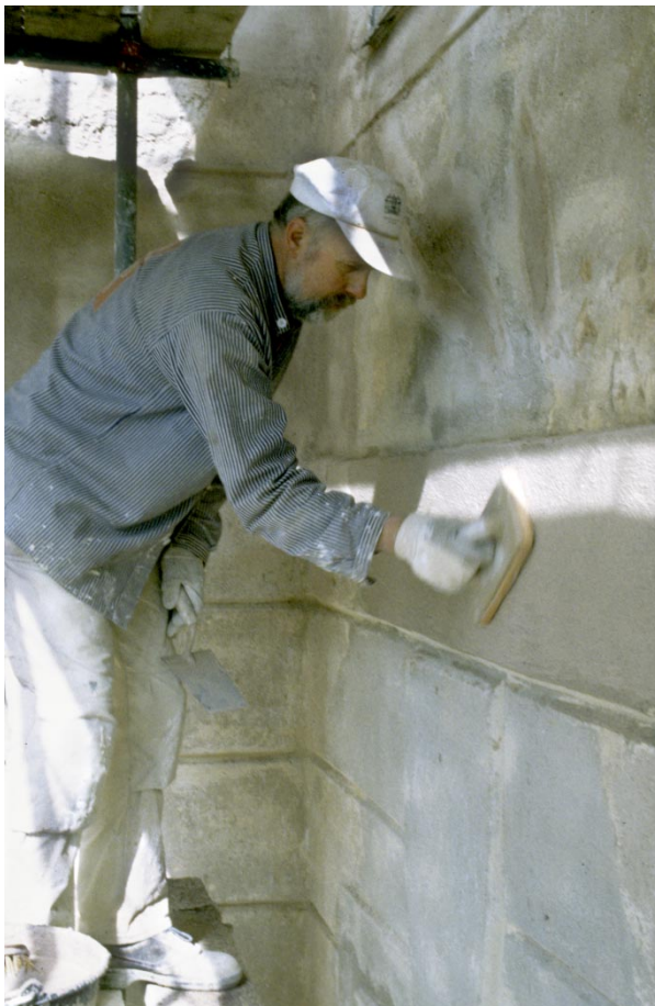
Plastering with lime at Mälsåker manor, Sweden. Photo Hans Sandström.
