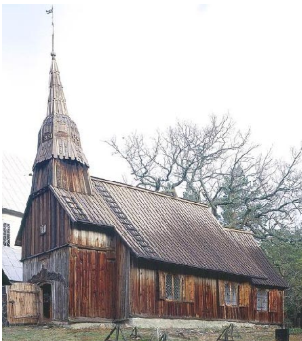
The wooden church from 1643 on the island Ruhnu, Estonia, has always been entirely tarred. Photo Peeter Säre.
