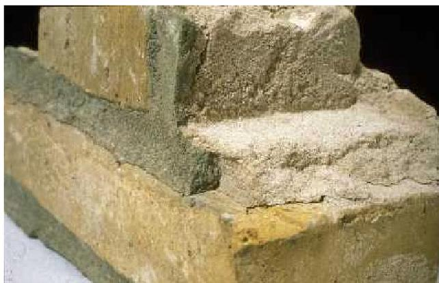
Part of a brick wall from the 1920s with lime mortar in bed and cross joints and a coloured decorative joint at the surface. Sweden. Photo Ewa Sandström Malinowski.
